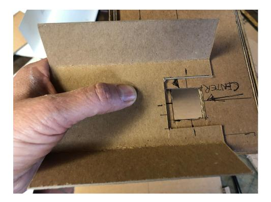
18. Glue the tray in place so the lens openings match up and secure your camera using a rubber band. The sides should compress a bit to hold everything in place.
